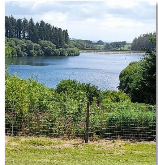
Elsewhere, as here at Wistlandpound, the original concrete post and wire boundary fence is being reinstated. The rebuilt line will run in the cutting beyond the new fence.
